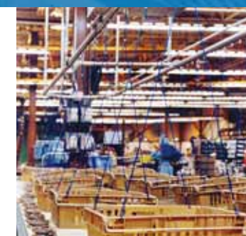
Small motor components transported in suspended baskets or totes on C-250 overhead conveyor.
